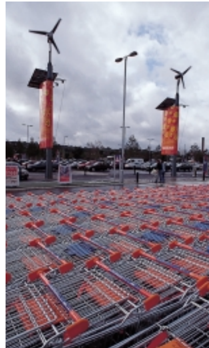
Wind-driven generators at Sainsbury's, Greenwich Peninsula
